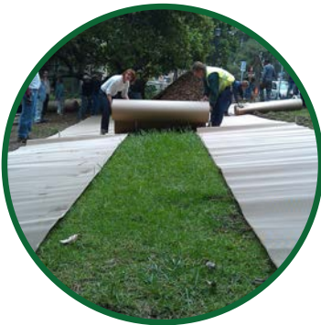
1. Site Preparation & Cardboard Sheet Installation
