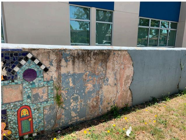
To repair and preserve this wall, loose material was scraped off and concrete adhesive was applied to the larger cracks. The wall was then primed and painted. A section of wall on the playground that was not treated during construction was also repaired and painted.
