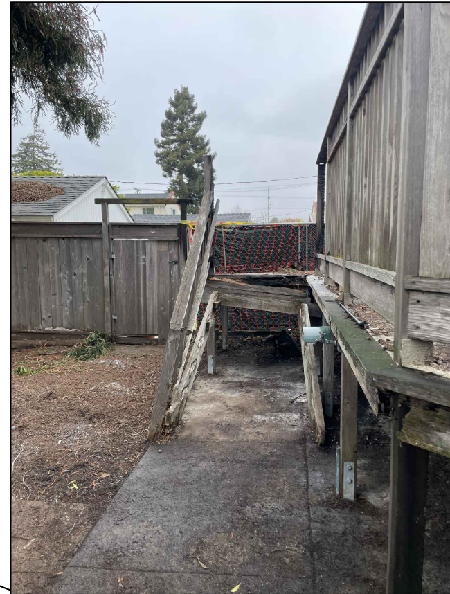
REPLACE FIRE-DAMAGED REDWOOD FENCE LIKE-FOR-LIKE
