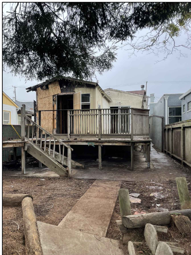
BACK OF HOUSE - REMOVE UN-PERMITTED LAUNDRY ROOM, ADD PRIMARY BEDROOM SUITE & 4TH BEDROOM, MATCH (E) STUCCO, ROOF, WINDOWS, DOORS & TRIM
